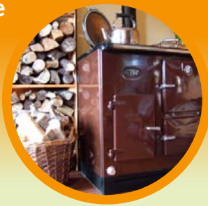
Large Log Fired Cooker and Back Boiler
